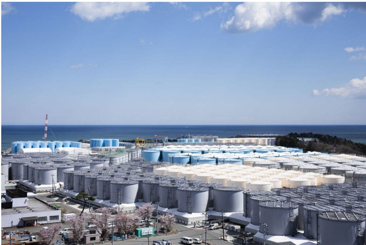
Fig. I-4. Storage tanks of ALPS treated water at FDNPS (Source: Website of Tokyo Electric Power Company Holdings, Inc.).
